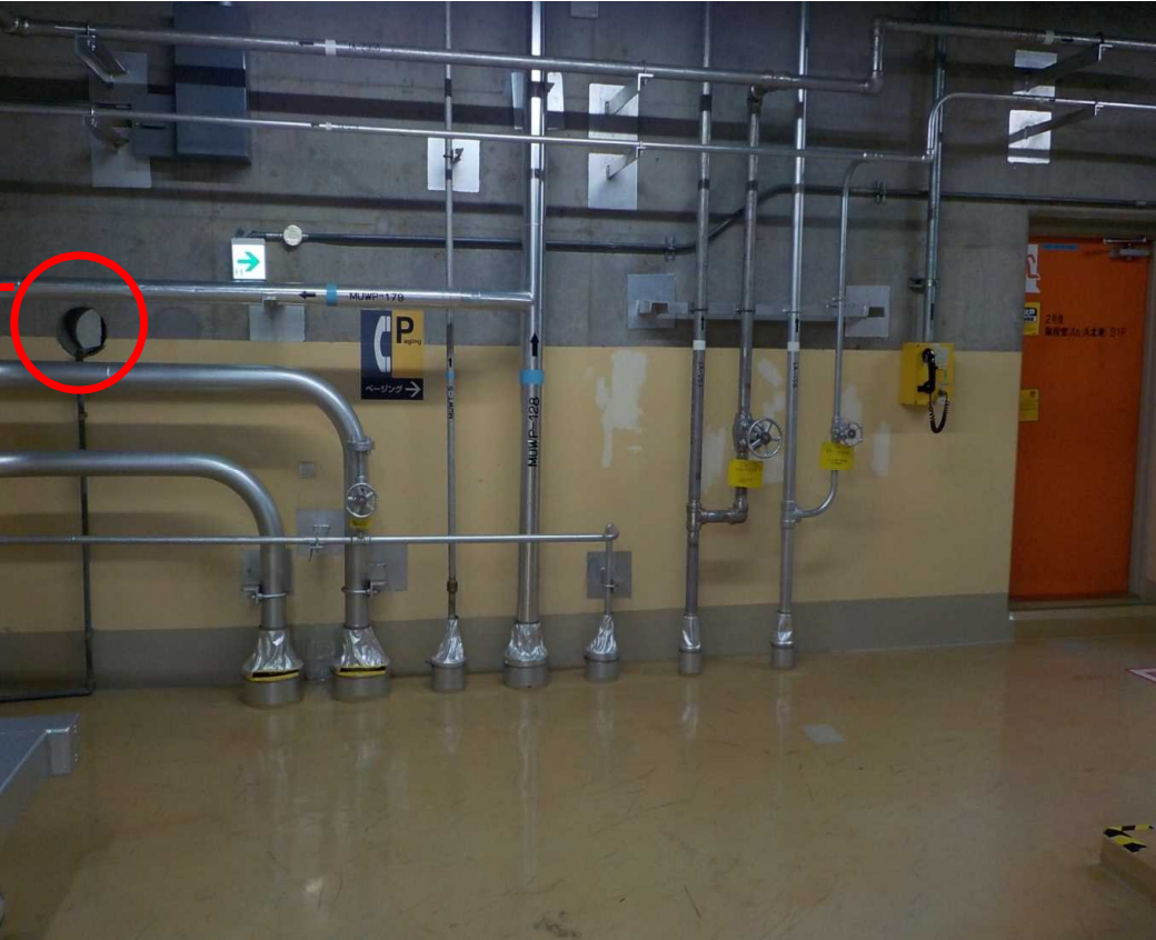
地下1階北東廊下側
