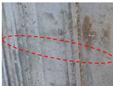
ひび割れ状況例 (No.1杭)
