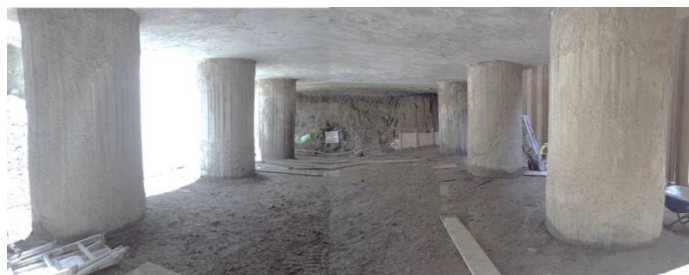
ひび割れ状況例 (No.1杭)
